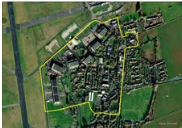
Brownfield land at Dalton Barracks
